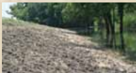
Mississippi Levee Board Damage estimate by Pimentel 2007.
